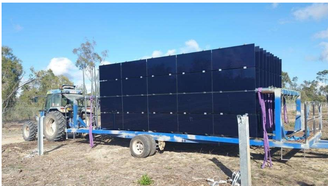
Figure 1: Trailer load of pre-assembled arrays delivered to the field
