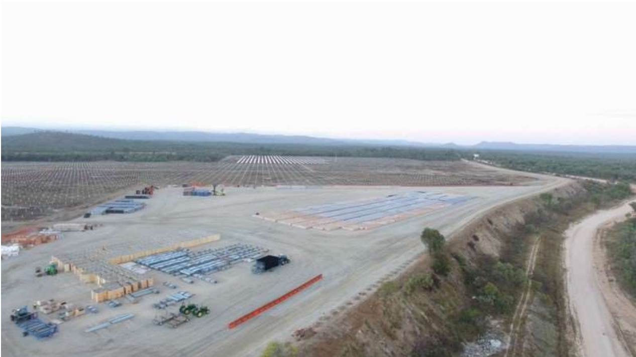
Figure 7: Aerial view of panels and lay-down site area
