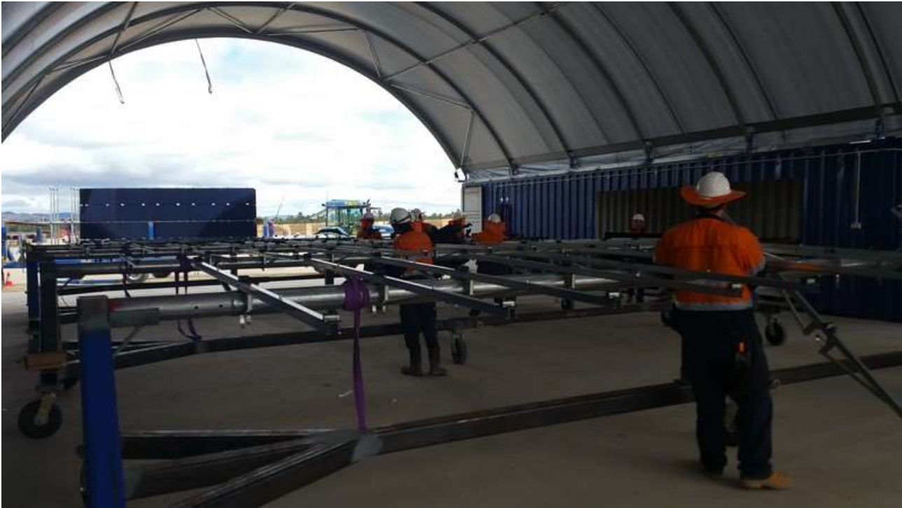
Figure 5: Solar panel installation workshop on site
