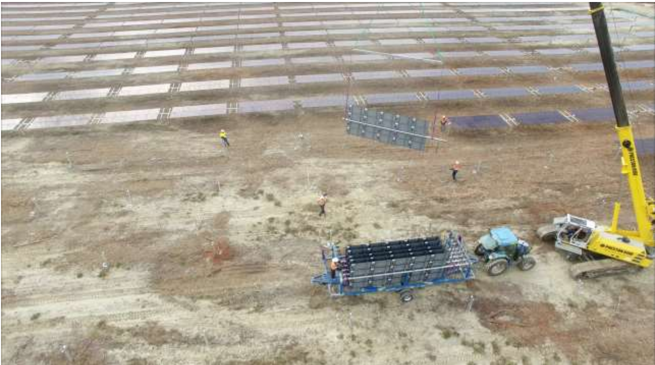
Figure 3: Solar module installation
