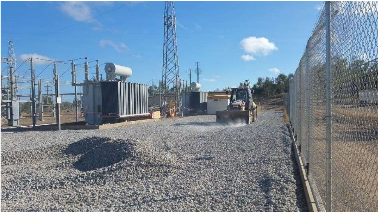
Figure 6: Final switchyard works
