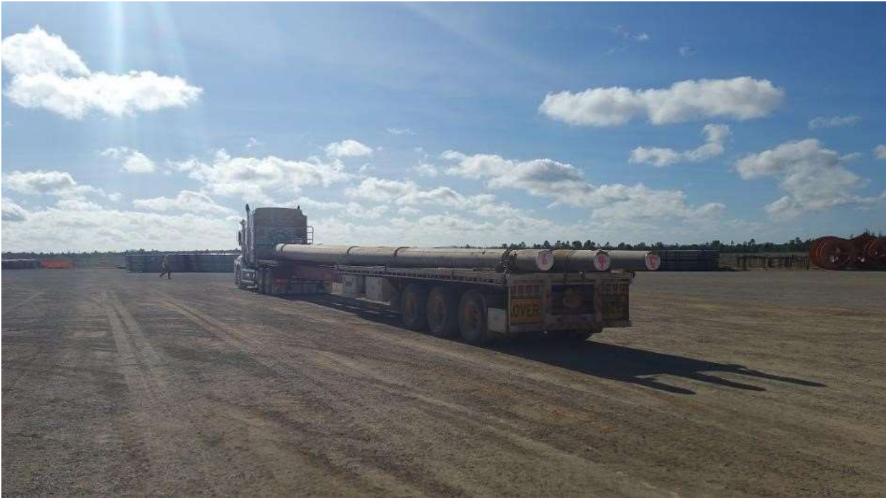
Figure 4: Power poles arriving on site
