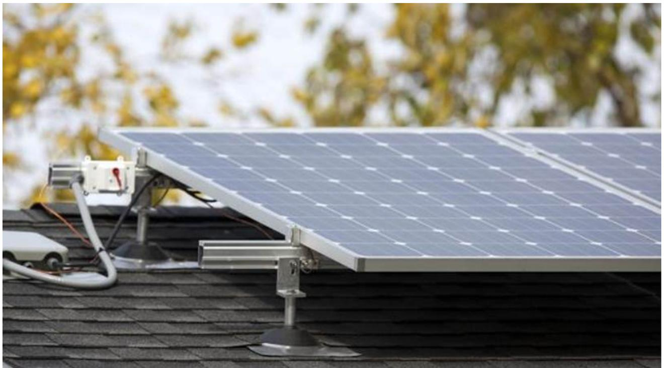
Photovoltaic cells on roof.
