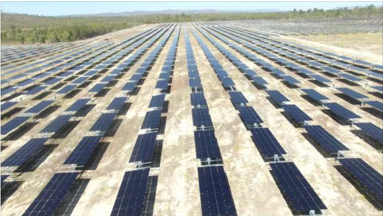
Figure 2: Continued installation of photovoltaic modules, pilings and trackers.
