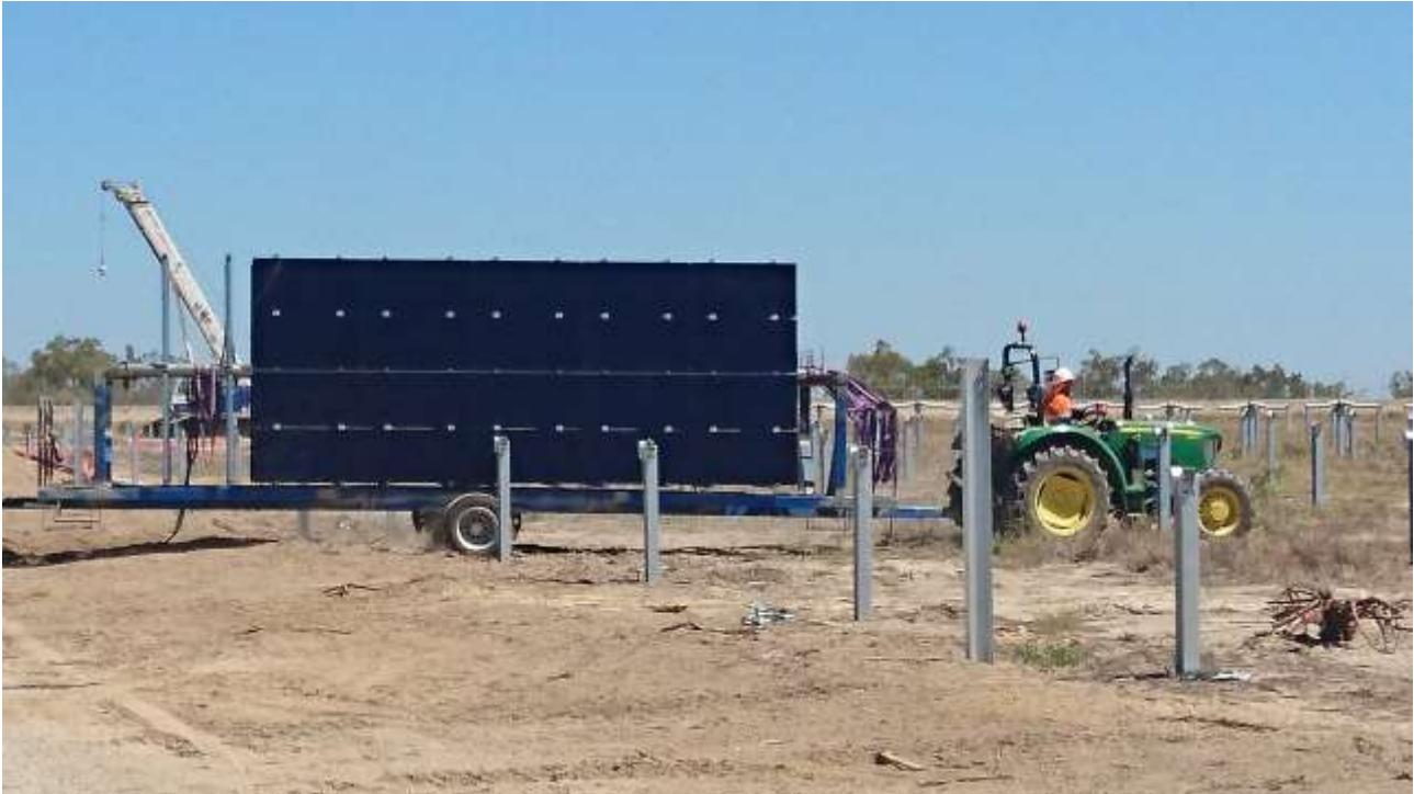
Figure 4: Tractor transporting modules to installation point.
