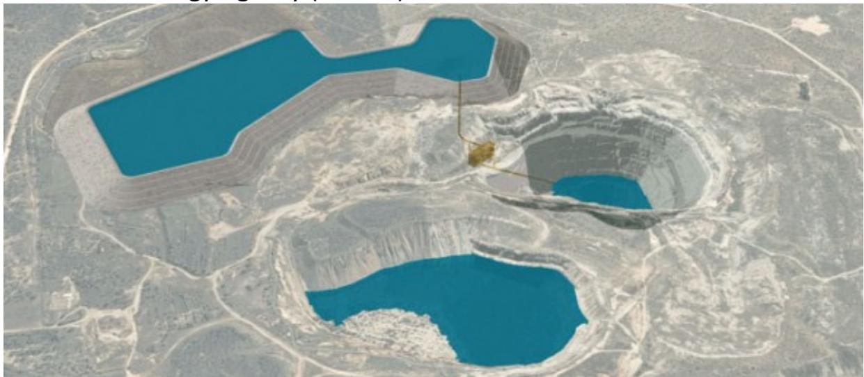
The “world first” project – which is being developed by NSW-based Genex Power – aims to transform two adjacent pits left over from the disused mine into a large-scale hydroelectric power plant, that will store excess generation from a 150MW solar array, and then sell it to the grid at times of peak demand.
