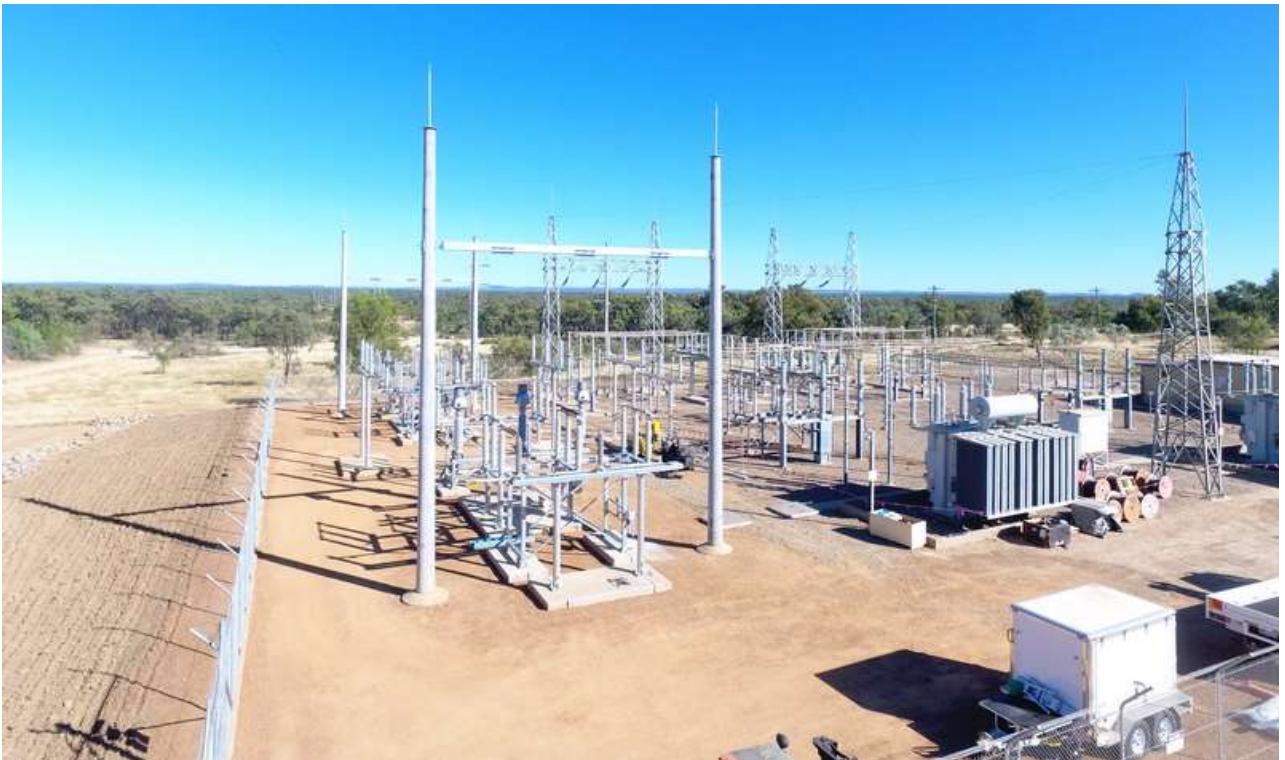
Figure 3: Ergon-Kidston Substation 75% complete.
