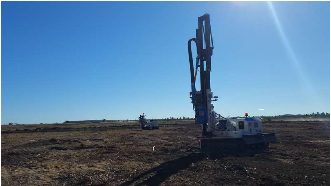
Figure 2: Piling rigs mobilised to site ahead of pile delivery.
