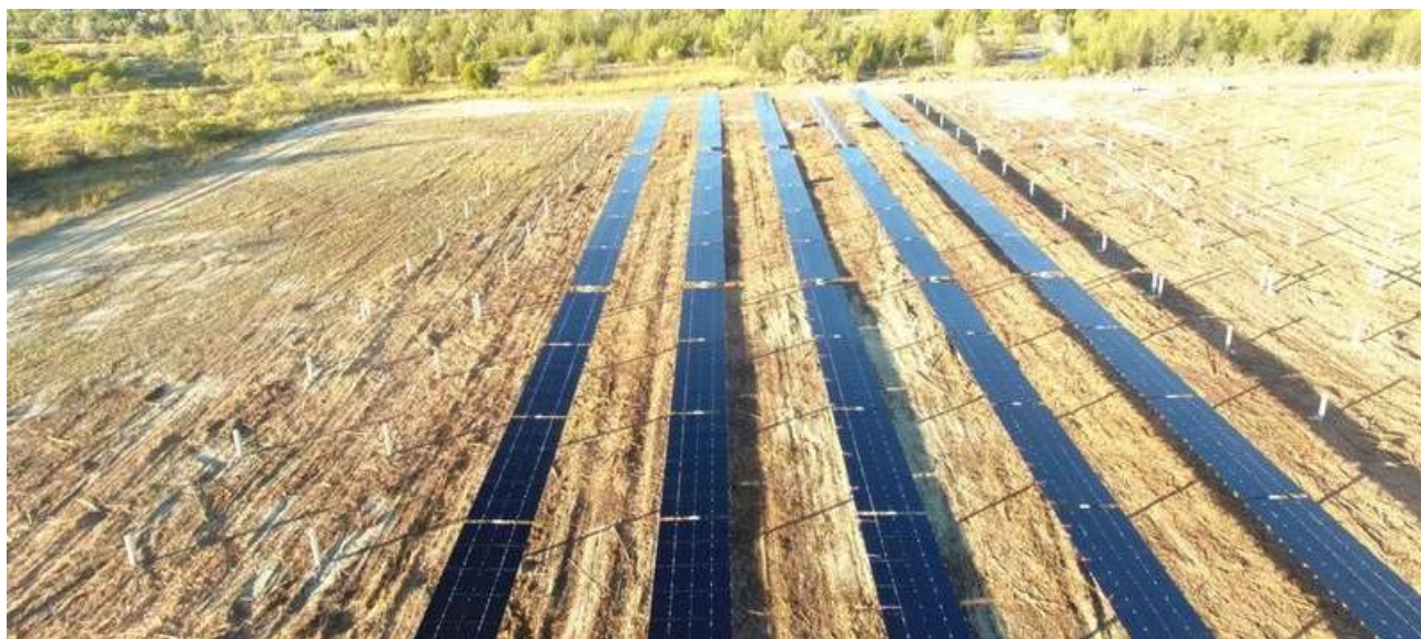
Figure 1: Aerial view showing progressive installation of solar panels
