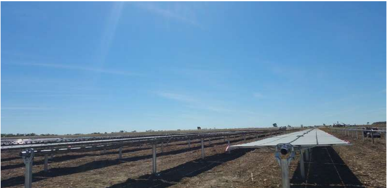
Figure 2: Solar panel installation showing poles and frames
