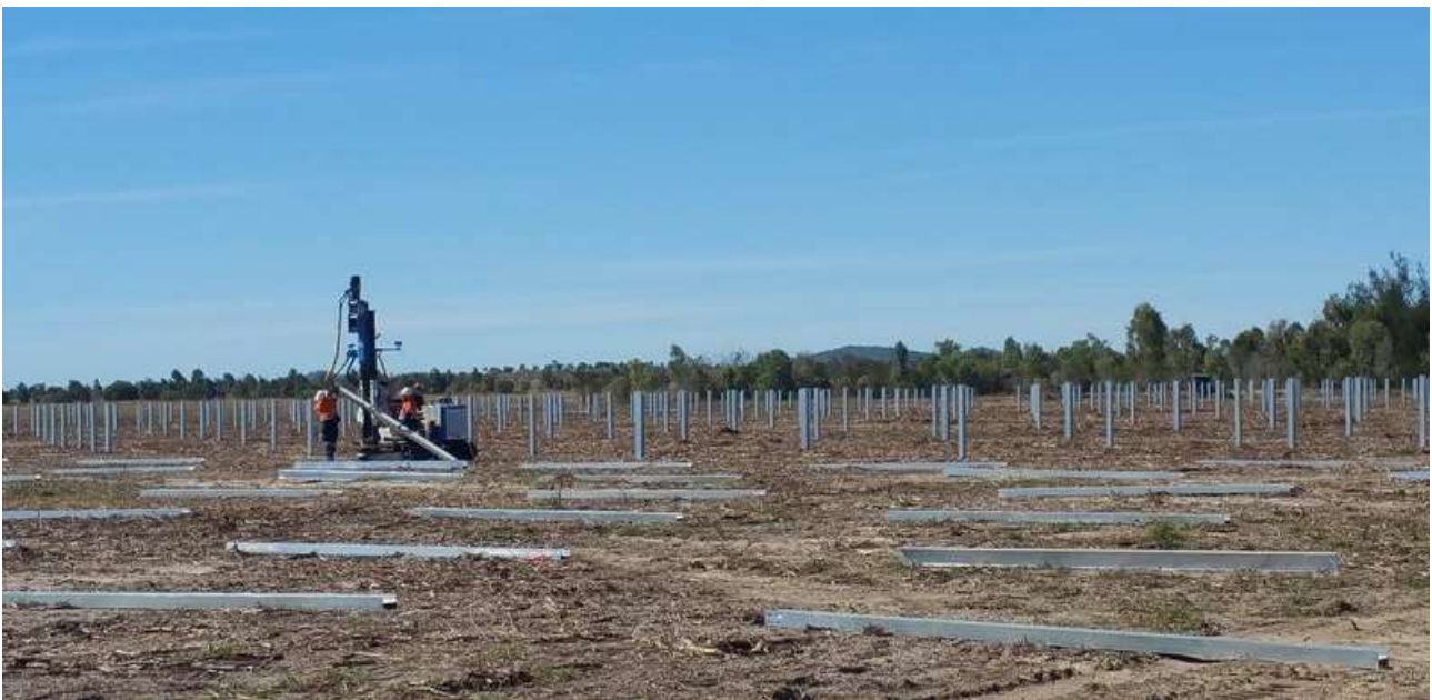
Figure 3: Piling rig in operation
