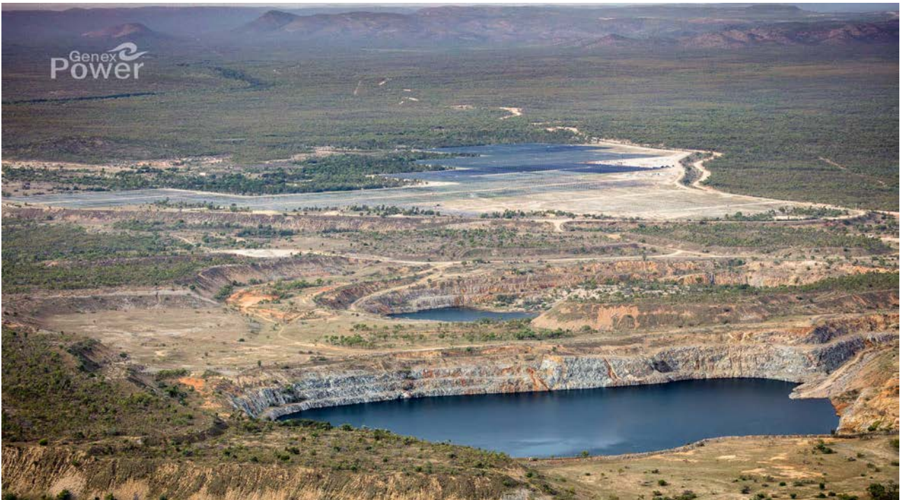
Figure 1: Kidston Renewable Energy Hub (photo taken in 2017 during construction of KS1).
