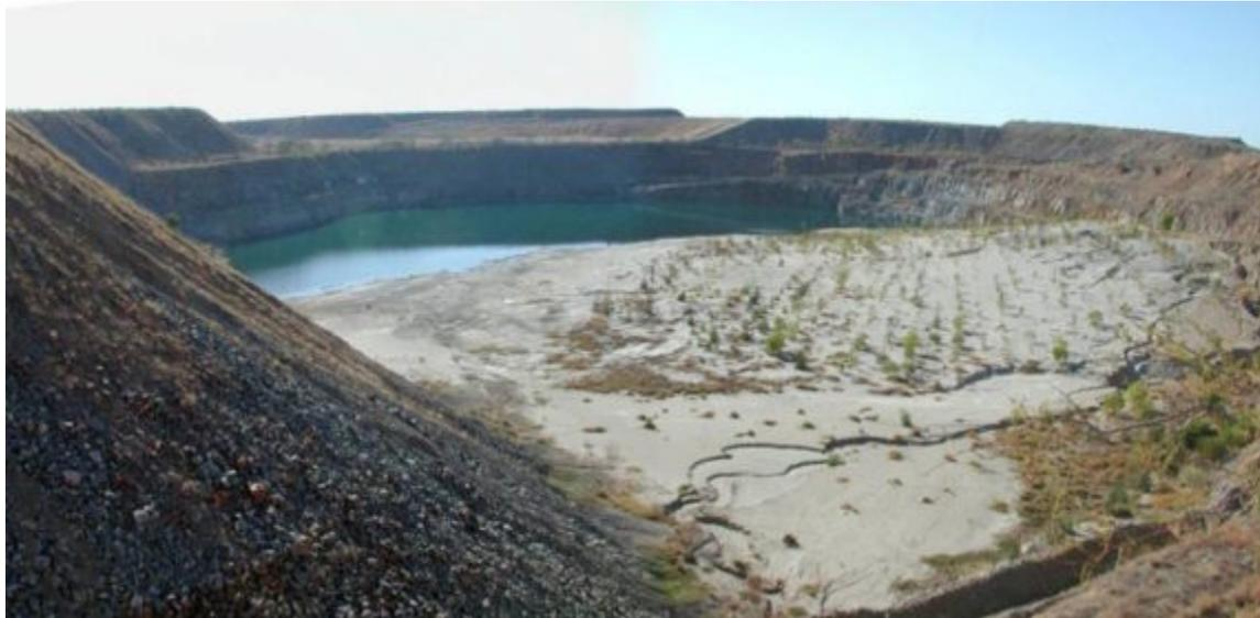
Australia's Genex Power is recycling a disused gold mine as a 400-[450 MW](#) pumped hydro storage project, with the potential to store and generate around 2,225 MWh daily, making this Australia's largest energy storage project by far.
