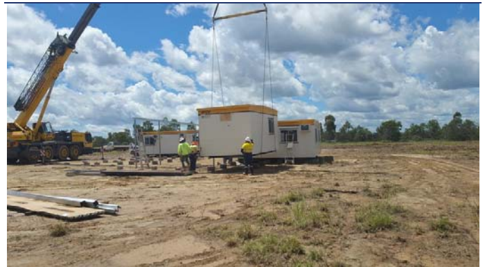
FIG.24: INSTALLATION OF SITE OFFICES – MARCH 2017
