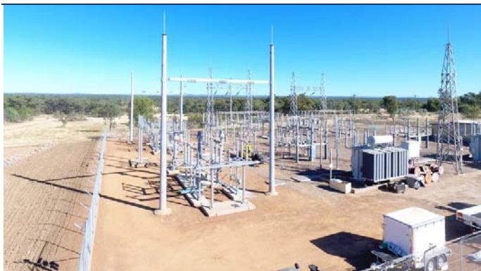
FIG.21: ERGON-KIDSTON SUBSTATION WORKS – MAY 2017
