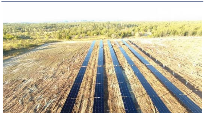
FIG.22: FIRST SOLAR PANELS INSTALLED – JUNE 2017
