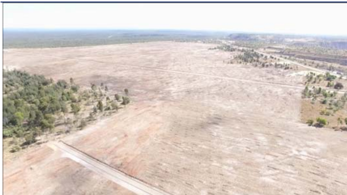
FIG.23: SITE CLEARING COMPLETE – MAY 2017
