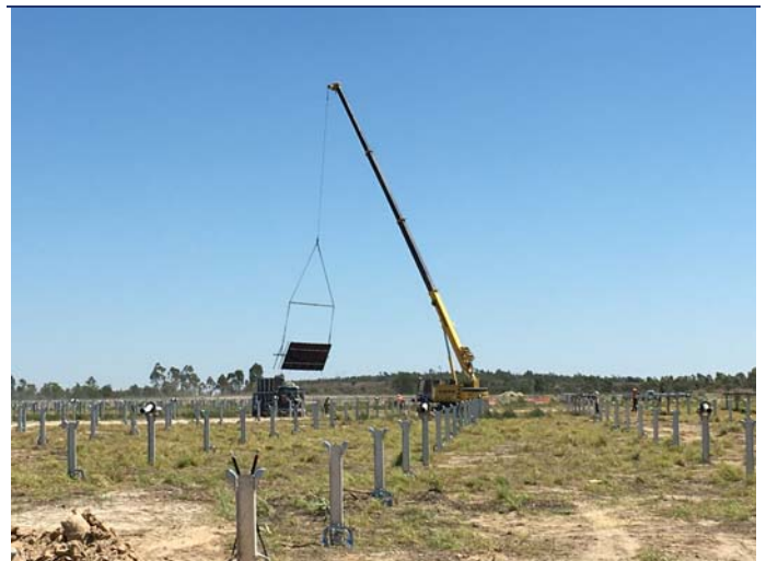
FIG.4: INSTALLING SOLAR PANELS
