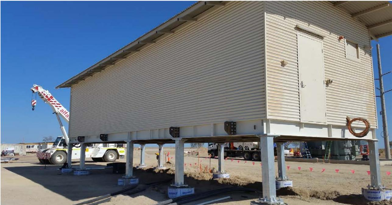
**Figure 3:** Installation of control room.
