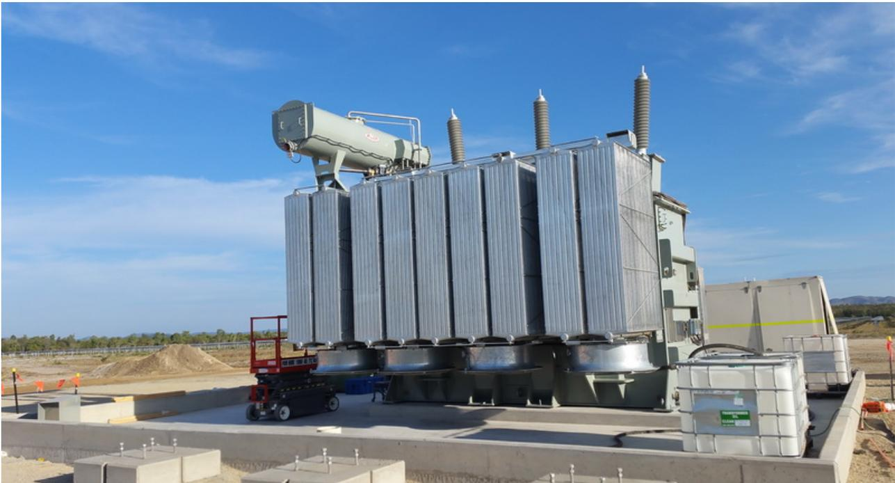
**Figure 2:** Installation of transformer.
