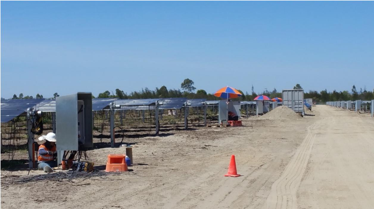
**Figure 5:** Electrical technicians terminating cables at the combiner boxes.
