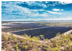
NOW EARNING: Genex Power's Kidston solar project.
